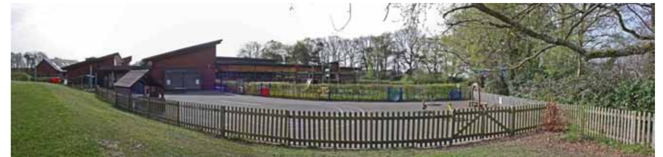
View to south west towards the school and play area.
